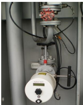
Obr. 2: Hydran senzor
