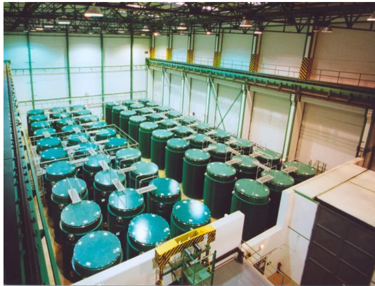
Fig. 2.14: Dry storage in Dukovany NPP, Czech Republic [23].
