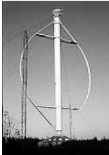
Fig. 2 Eole C, a 4200 kW Vertical axis Darrieus wind turbine with 100 m rotor diameter at Cap Chat, Québec, Canada.
