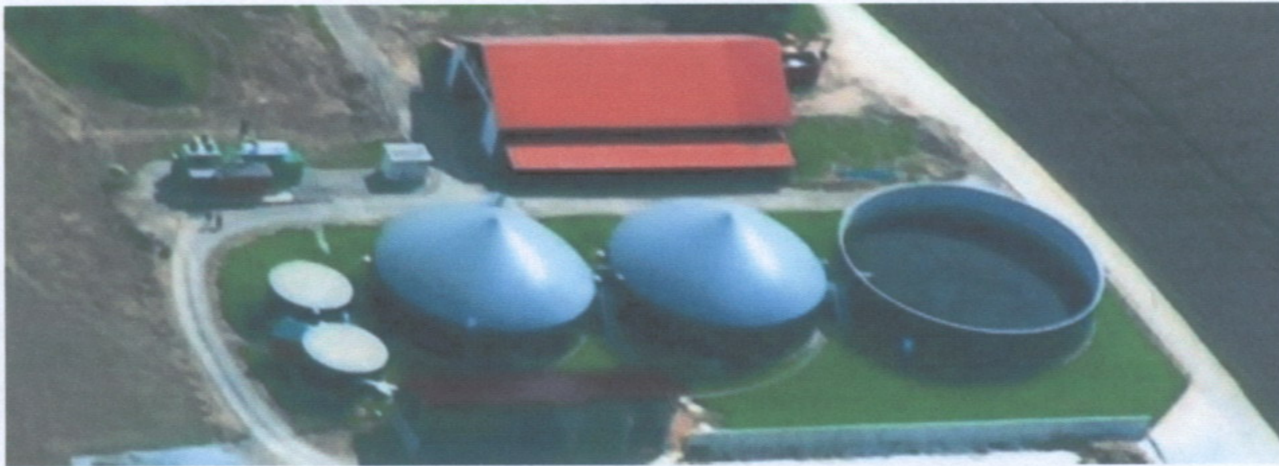
Figure 3: Technological buildings of the biogas station
