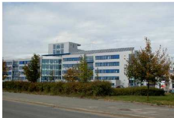
Fig. 10.: 20kWp photovoltaic system
