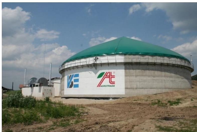
Figure 2 – The actual view at biogas power station in Rozhanovce
